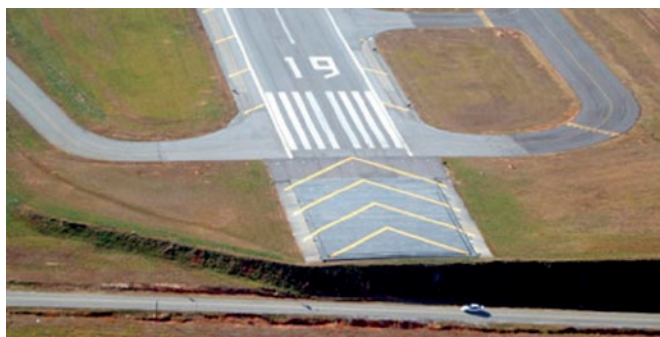
Figure 9.1—Photograph of an EMAS Installation
