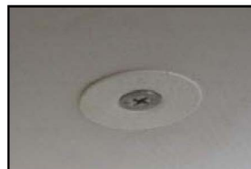
EXAMPLE OF CORRECTLY INSTALLED FASTENER ELEMENT
