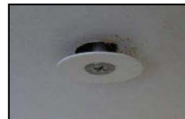
EXAMPLE OF LOOSENED FASTENER ELEMENT
